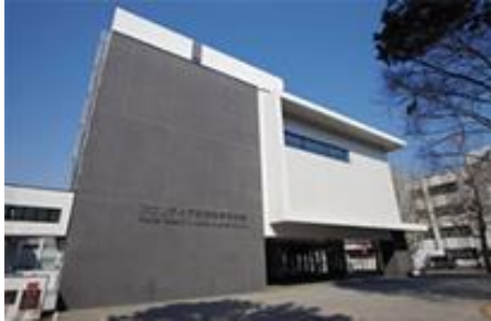
Frontier Research in Applied Sciences Building
